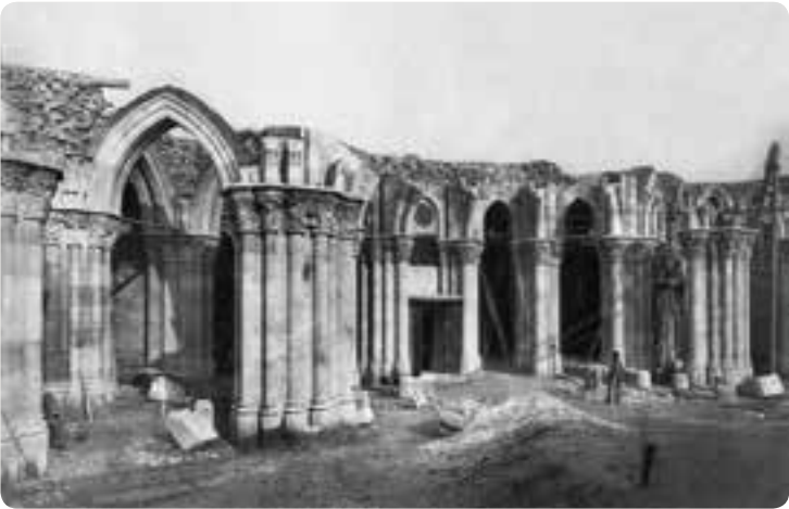
Photograph of the crypt in construction published in 1886.
